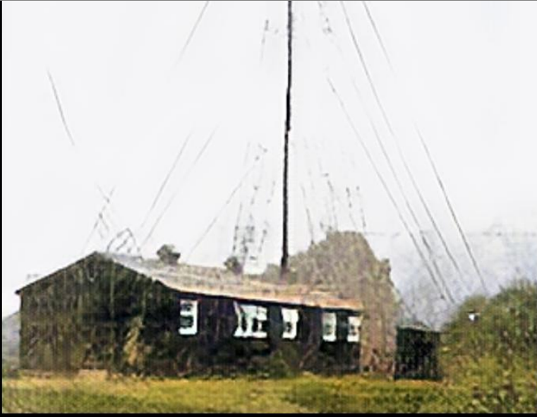
The transmitting hut and aerial of the Dublin broadcasting station. Dublin has a power of 14 kw., and transmits on a wave-length of 413 metres.
